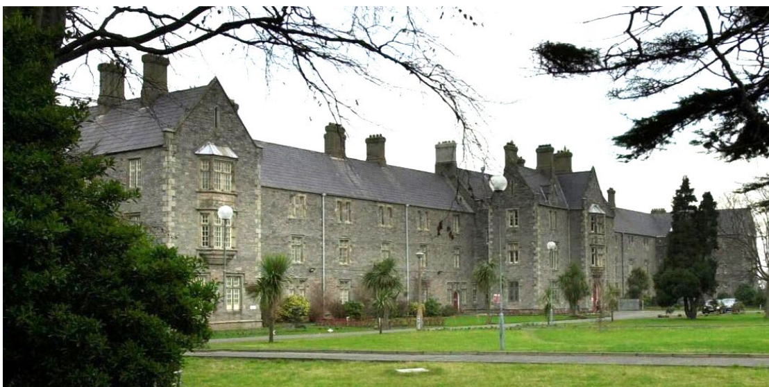
Figure 15.11: Main Hospital Building.
