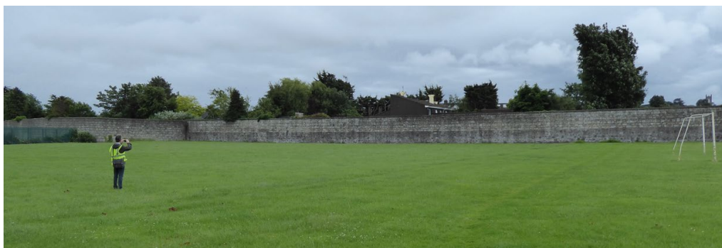
Figure 15.14: Internal face of Perimeter Wall to west of the Site.
