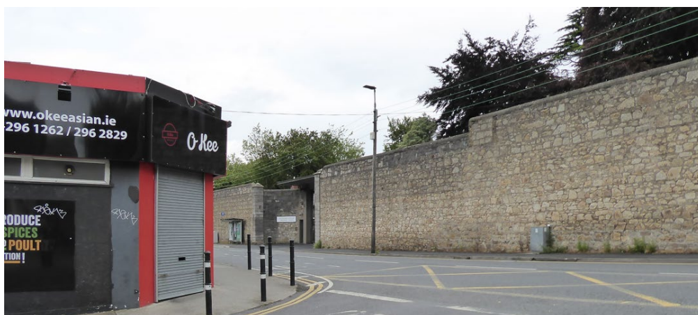
Figure 15.13: Perimeter Wall and Entrance on Dundrum Road.
